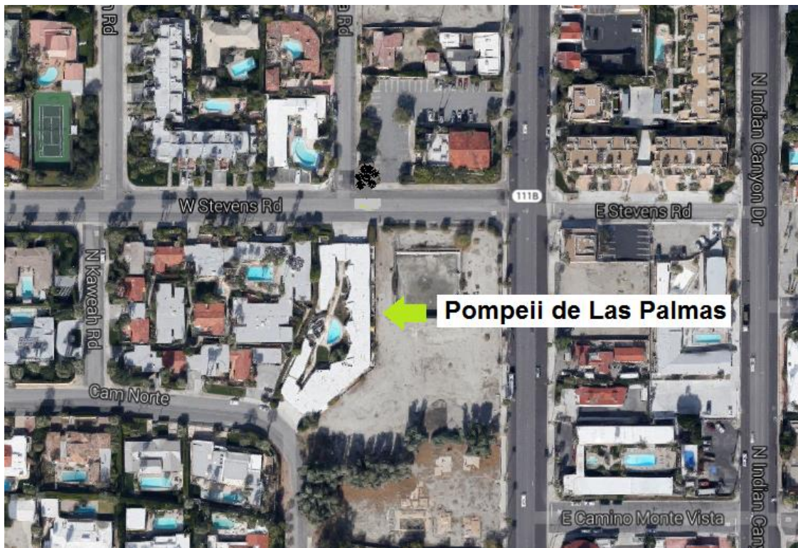
Aerial view of Pompeii de Las Palmas complex (oriented north)
